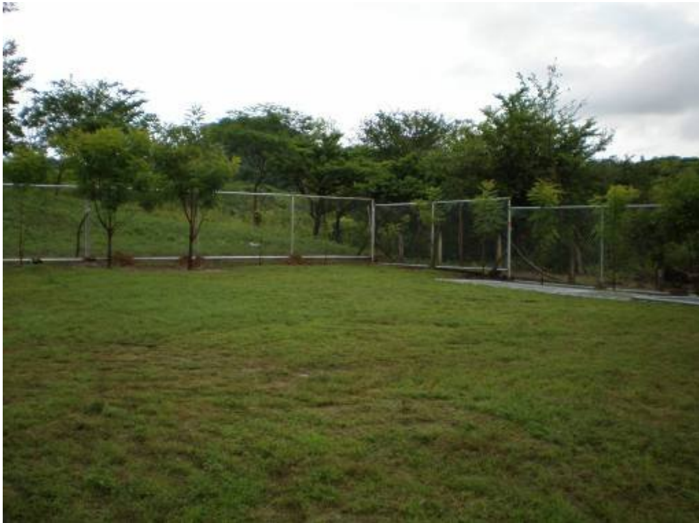
9- The fence already installed in the yard of the School.
