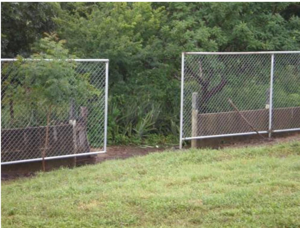
8- Front entrance of the Osneida School with the fence now installed.
